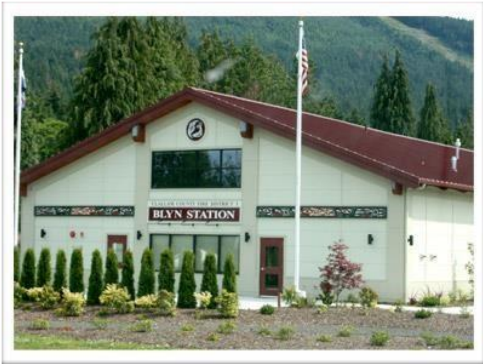
Clallam County Fire District 3 Station in Blyn
