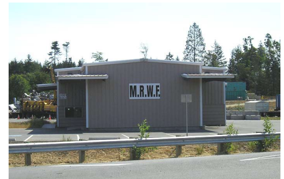
Moderate Risk Waste Facility
